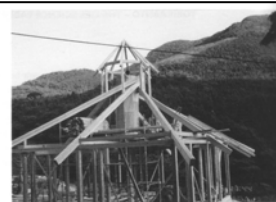
▲ 8.20 The RF structure becomes stable when all the beams are installed. (Photo: Yoichi Kan.)
